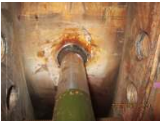
4) Continue full weld and test until as above photo.
