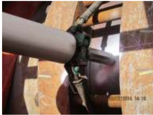
2) Mark and tag weld location of TDs. Ensure full contact at tip on tube sheet.
