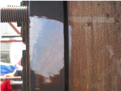
1) Grind off rust or paint.
