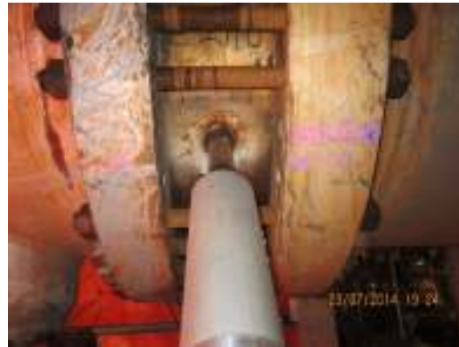
3) Weld all round the tip of TD. Check with non destructive penetration test for good welding.
